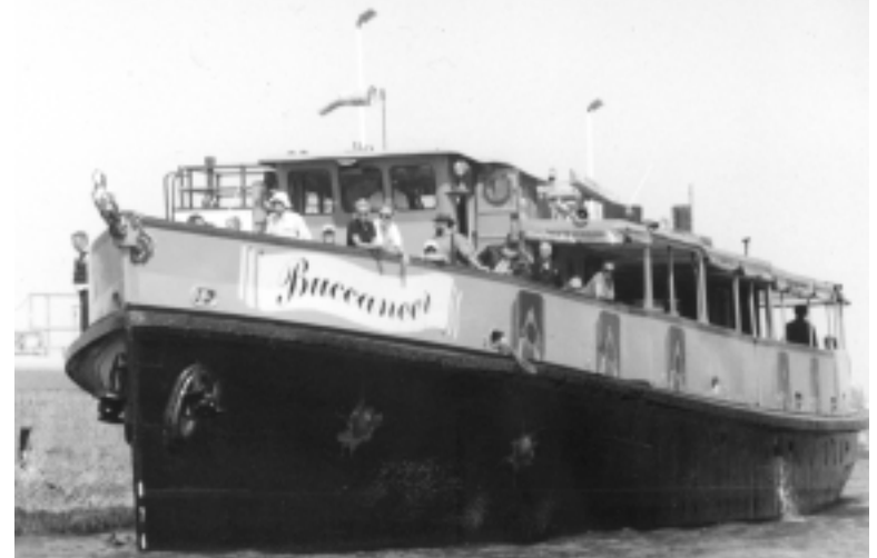
The Buccaneer , formerly the US Coast Guard ship Dexter , in May, 2000, when she carried tourists to view the scuttling of the Holly barge off Chicago. Plans are to scuttle the Buccaneer off Chicago by late 2008. The steel housing, welded onto the hull, will not be torn off by the sinking, making it a more interesting scuba dive site. The mermaid figurehead, added in the 1990's, has been stolen from the ship, which awaits clean-up and legal permission for the scuttling. Photo by Cris Kohl
